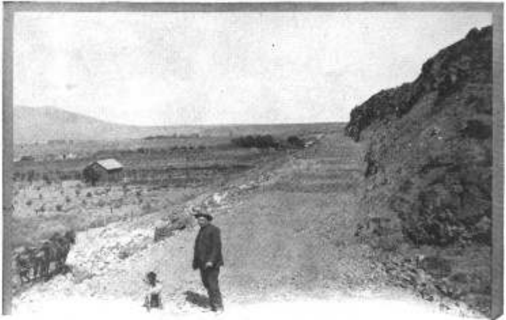
PART OF THE NORTH COAST ROAD-BED. No expense has been spared to prepare the way for the track.
