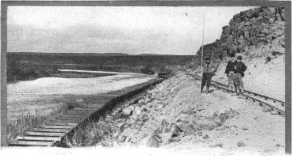
CANAL MOVED TO MAKE ROOM FOR RAILROAD TRACKS. Fifteen miles of the Kiona Canal were purchased for this purpose.
